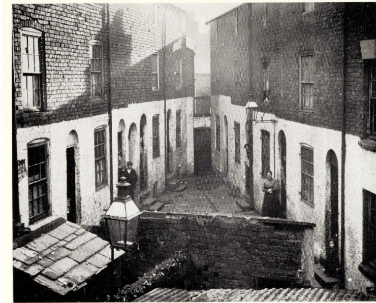
A TRIANGULAR SHAPED COURT, WITH TUNNEL ENTRANCE, CONTAINING NINE INSANITARY HOUSES, BACK TO BACK WITH ADJACENT FRONT HOUSES.
