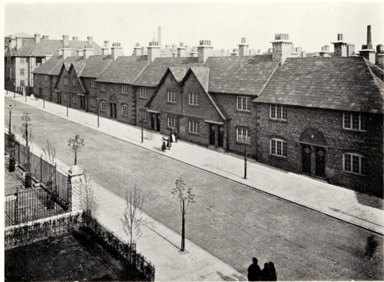
A VIEW OF SELF-CONTAINED COTTAGES IN BEVINGTON STREET, LOOKING FROM TITCHFIELD STREET. Erected on the site of former insanitary property. (This Street was formerly only 28ft. wide, and is now 60ft. wide.)
